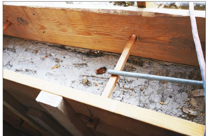
The method of pouring tabby for the Adam Strain Building is being replicated from the original tabby making process developed by Thomas Spalding, using one-foot boards spread apart and fastened with wooden pins.
