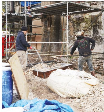
The method of pouring tabby for the Adam Strain Building is being replicated from the original tabby making process developed by Thomas Spalding, using one-foot boards spread apart and fastened with wooden pins.
